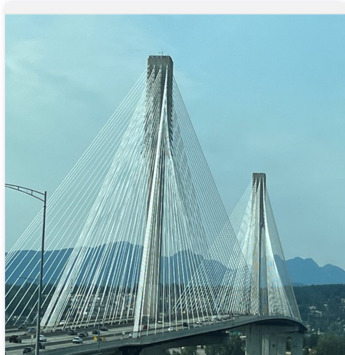
Port Mann Bridge, Vancouver BC
